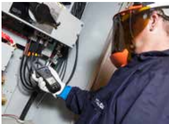
Analyze Power-related Issues
