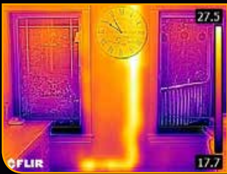
Pipe in wall Thermal Image with MSX
